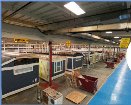
BUILD UNITS IN FACTORY
