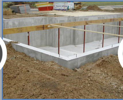
PREPARE FOUNDATION AT SITE
