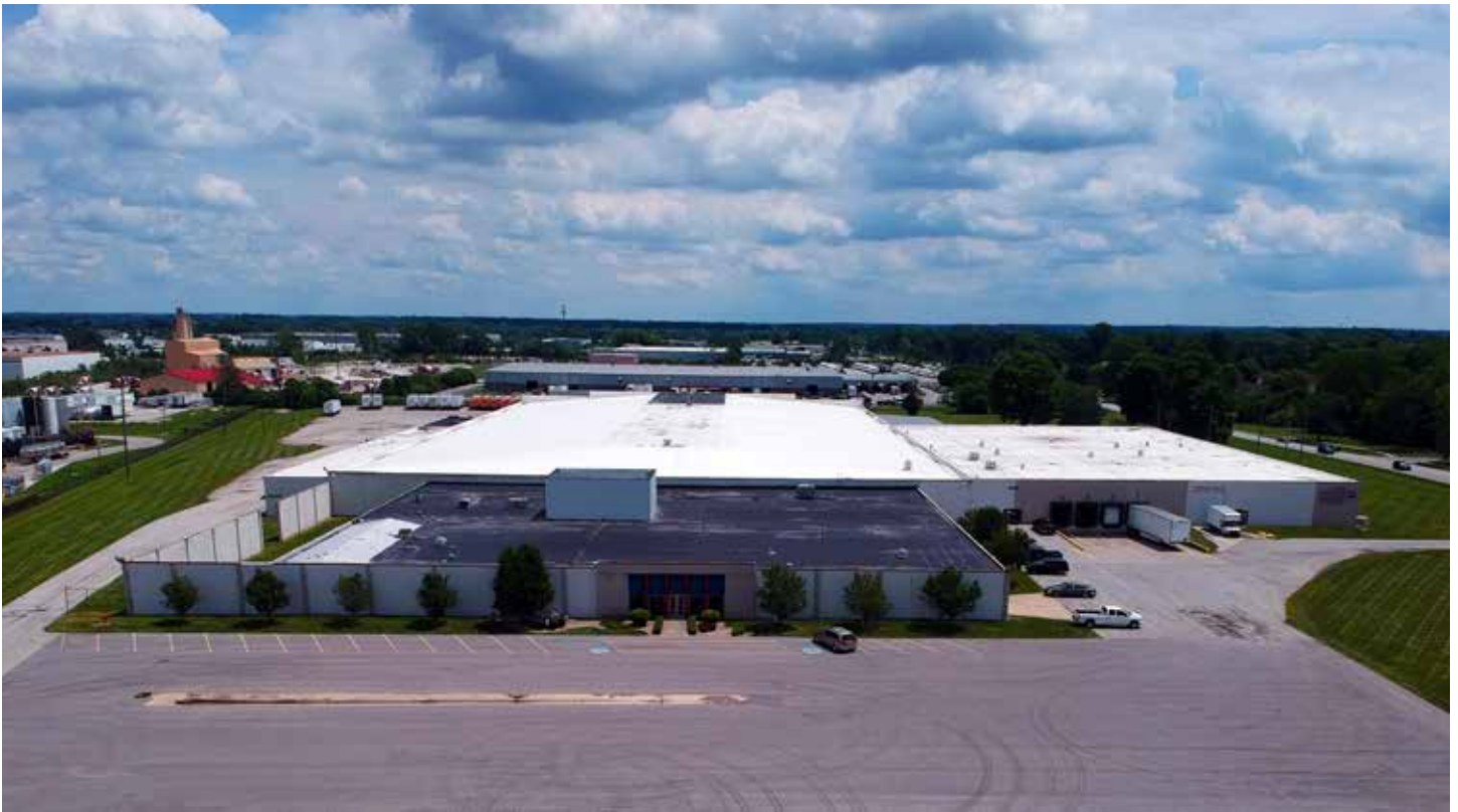
Volumod Factory, Indianapolis, Indiana
